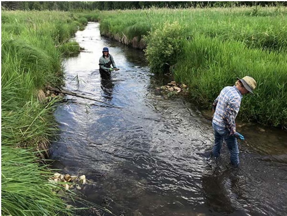
Don and Jo Harris were working in the creek rolling rocks out of the centre of the channel to the edge of the river. The creek will then become deeper, narrower and colder.
