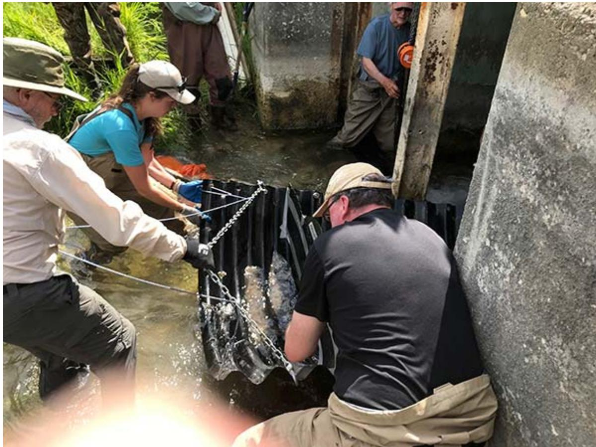
Moving the heavy culvert in place became more difficult when it filled with water
