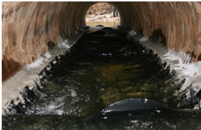
Looking downstream at the fish ladder grouted in place and running full. (Photo courtesy of CSPI)
